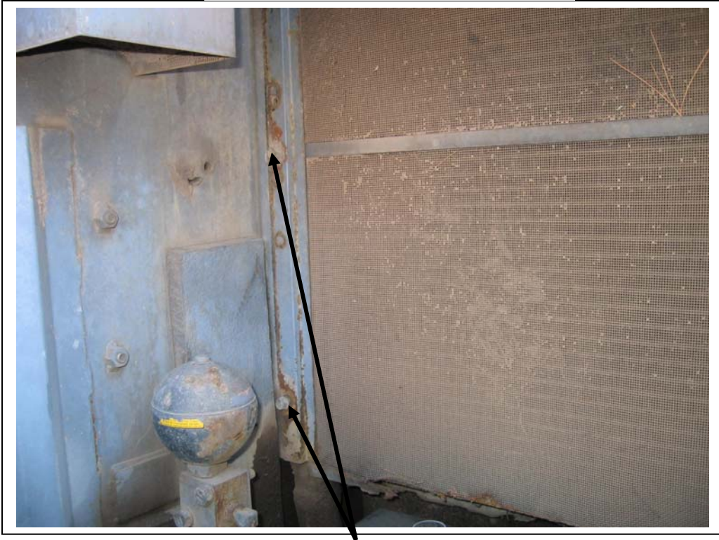
Use existing bolt holes to mount the condenser frame.
