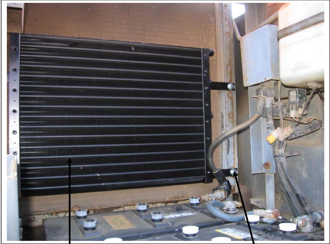
Condenser coil in place.
